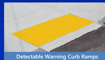
Detectable Warning Curb Ramps
